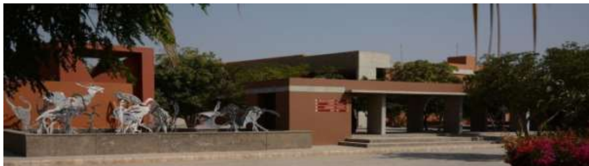
Fig. 7 Living, learning, design centre (LLDC) entrance view.
