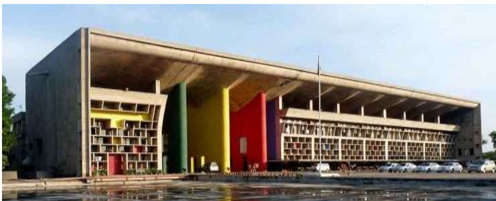
Fig. 2 View of The Capitol Complex, Chandigarh, India- expressing bold geometric shapes and structural elements.
